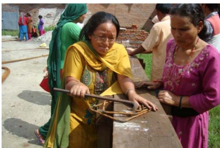
Photo 1. Female Masons Trained in Earthquake Safe Construction. Source: Kathmandu Metropolitan City and supported by the UNDP Comprehensive Disaster Risk Management programme. http://bit.ly/1FEDLUL
